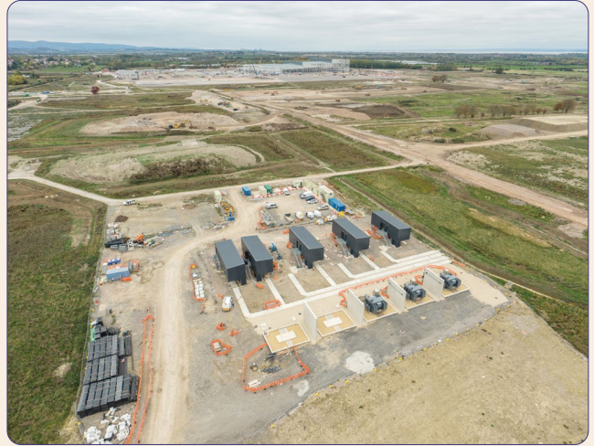
Interim power connections under construction
