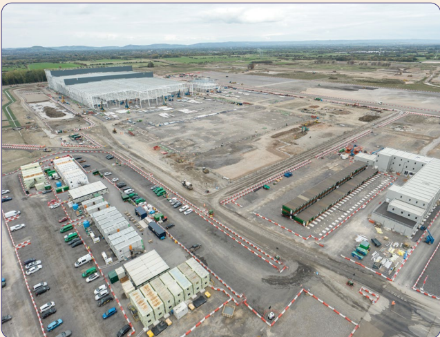
Installation of temporary site offices to the south of Building One
